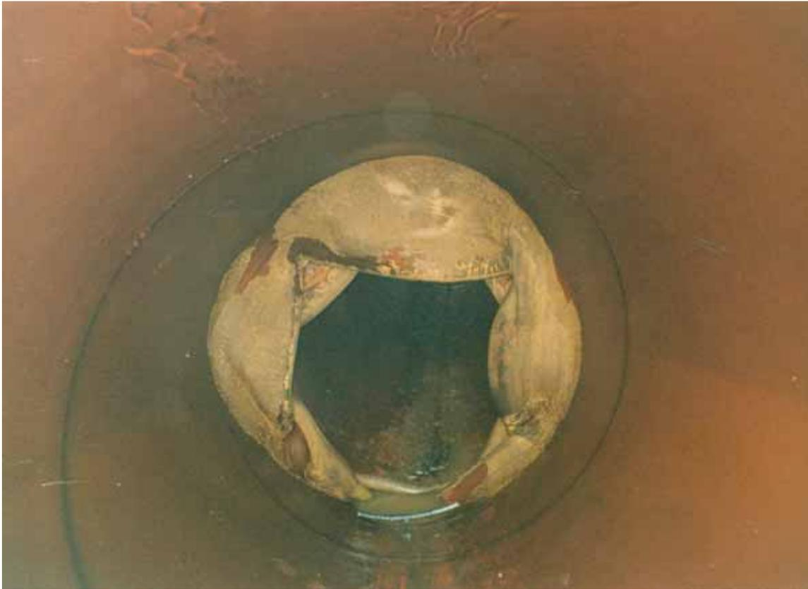
*Figure C7-2. Wrinkle of 2.2 Meter Diameter Thames Pipeline*
