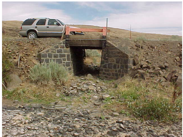
Figure 3. Outlet of Typical Short Span Bridge
