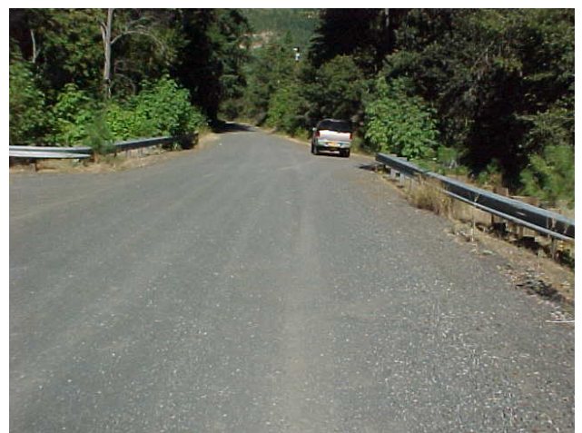
Figure 5. Bridge 65C65, Wilson Road over West Fork Mosier Creek
