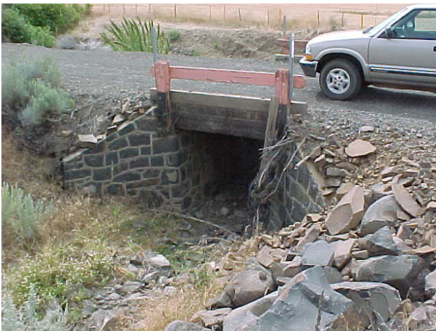
Figure 2. Inlet of Typical Short Span Bridge
