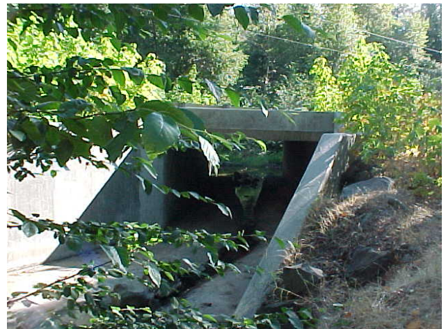
Figure 4. Inlet of Box Culvert, with Fish Passage Channel
