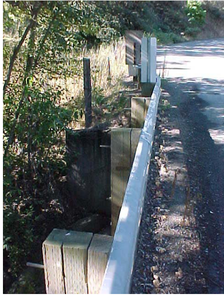
Figure 7. Wilson Road (constant width over bridge).
